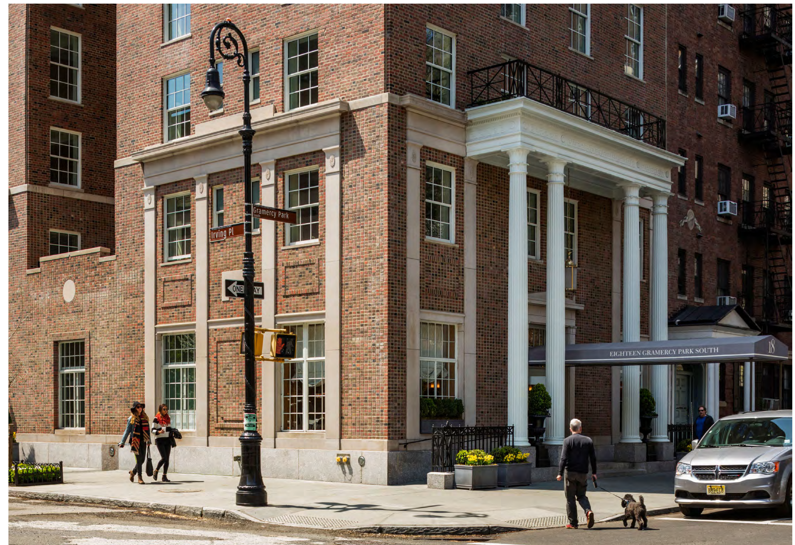
1. LOOKING SOUTH-WEST AT CORNER OF GRAMERCY PARK SOUTH AND IRVING PLACE
